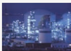
Refinery and petrochemicals
